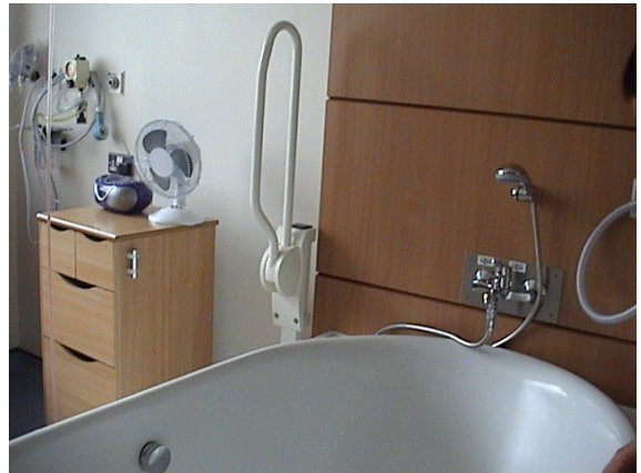
Photograph 13 Fold down grab handles to aid mother in and out of the pool
